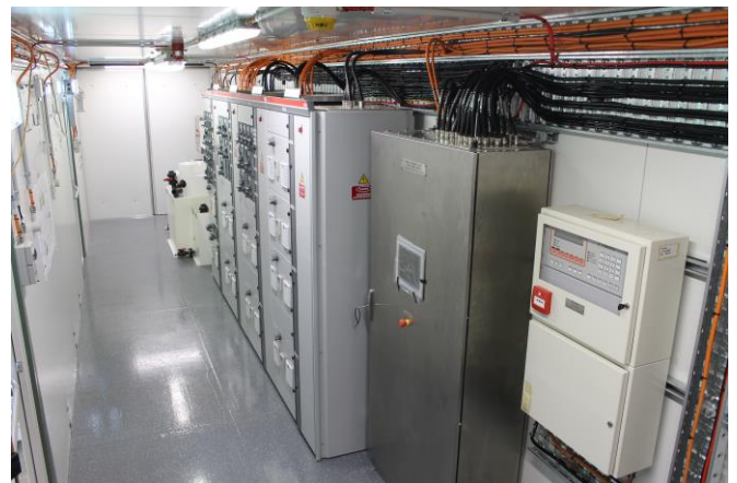
Containerised ancillary equipment and control system
