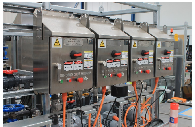
Pump motor controls. Signage in English and Mongolian.
