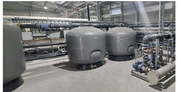
MAK Water skid mounted MMF plant
