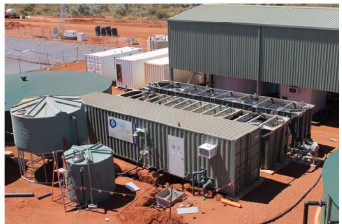
MBBR being installed onsite at the accommodation camp
