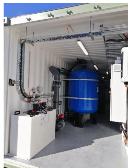
1,000 m 3 per day containerised Multimedia Filtration (MMF) plant with hypochlorite disinfection
