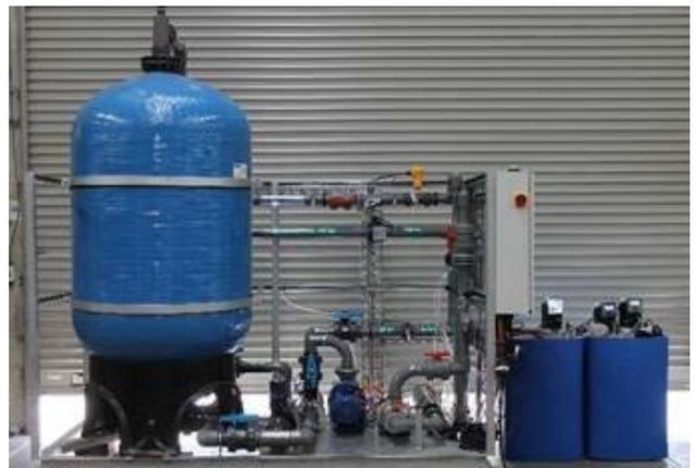
*Bore water treatment system for potable use*
