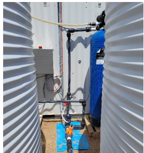
MAK Water MMF Pre-Treatment neatly installed between pilot plant container and balance tanks
