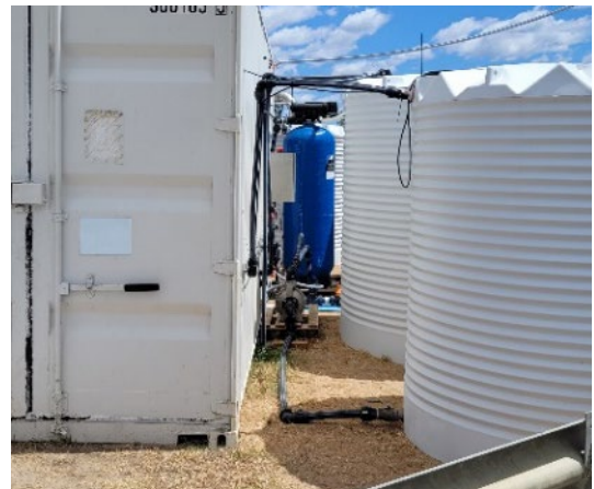
MAK Water MMF Pre-Treatment neatly installed between pilot plant container and balance tanks
