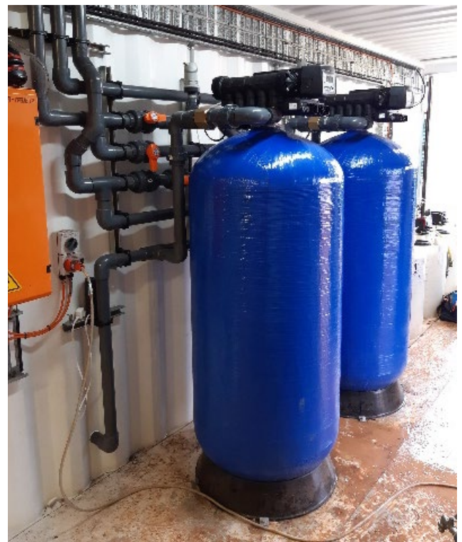
New MMF system during installation in the existing sewage treatment system
