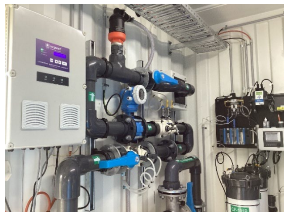
Internal view of the containerised MMF plant
