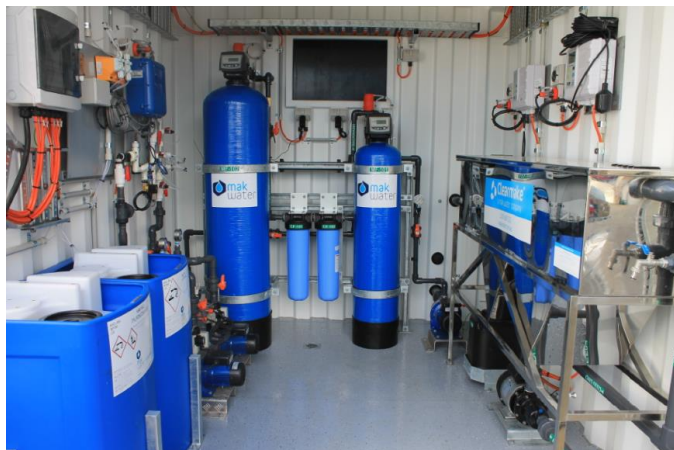
Water recycling system capable of treating 1,500 litres per hour of wash bay water
