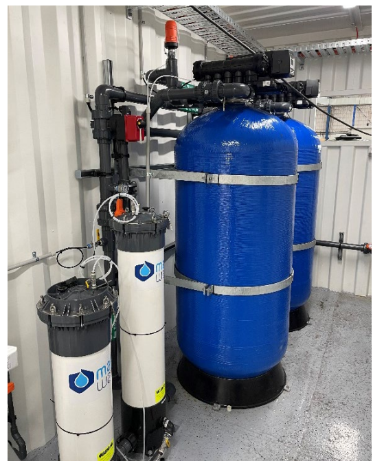
Inside the containerised MMF plant
