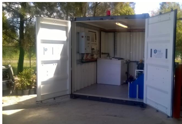
pH Adjustment Batch System capable of treating up to 1,000l/h of acid wastewater
