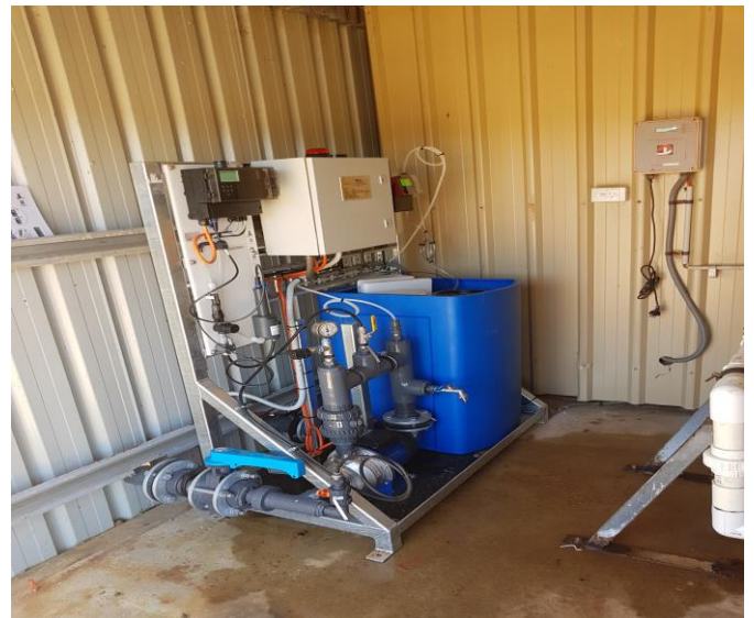
MAK Water installation of a SHDR system
