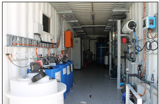
Internal view of the containerised SWRO plant
