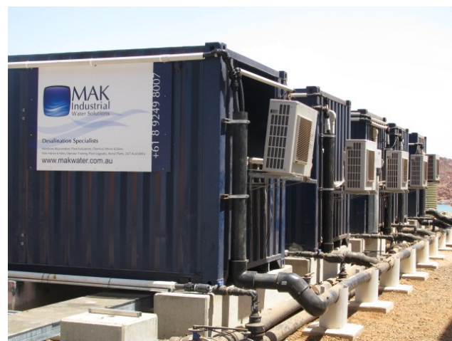
The RO Plant has a production capacity of 200,000l/d
