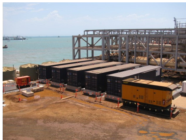
Five separate containerised RO Plants on site in Karratha
