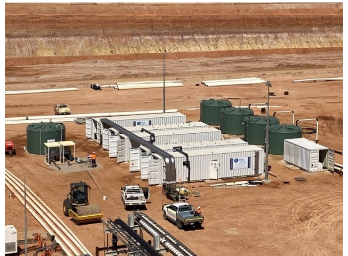
MAK Water containerised SWRO plant installed onsite
