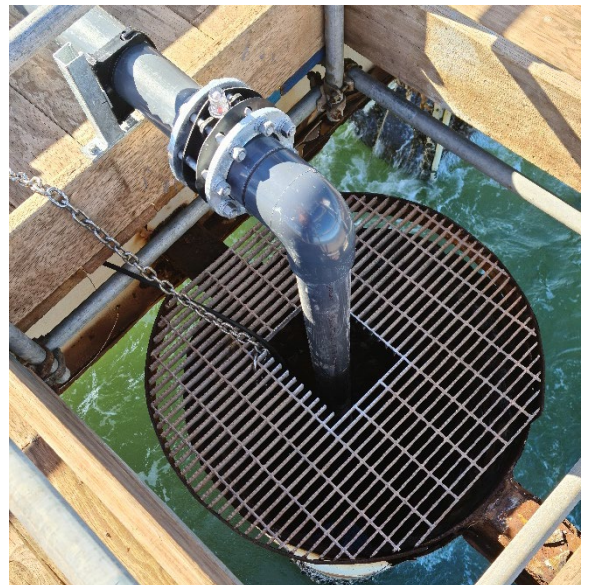
Custom seawater inlet design installed on existing jetty.
