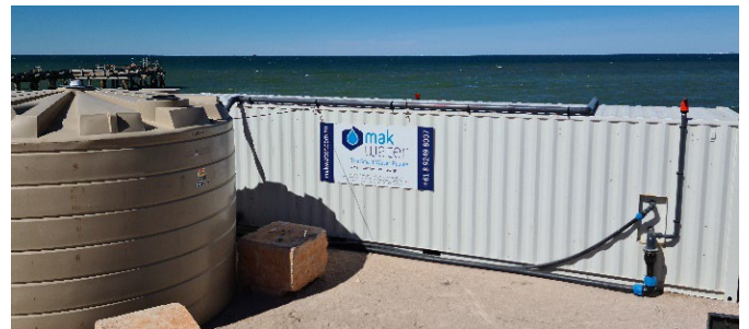
MAK Water containerised SWRO plant installed onsite
