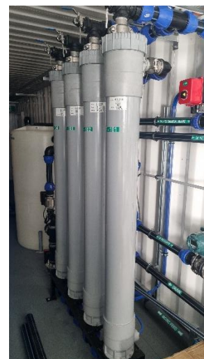
Internal view of the 300m 3 /day containerised UF plant
