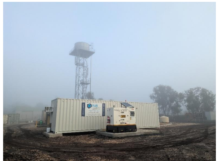
MAK Water containerised UF plant installed onsite
