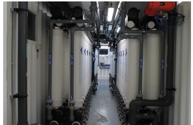
Containerised 5,300 m 3 /day Ultrafiltration (UF) plant
