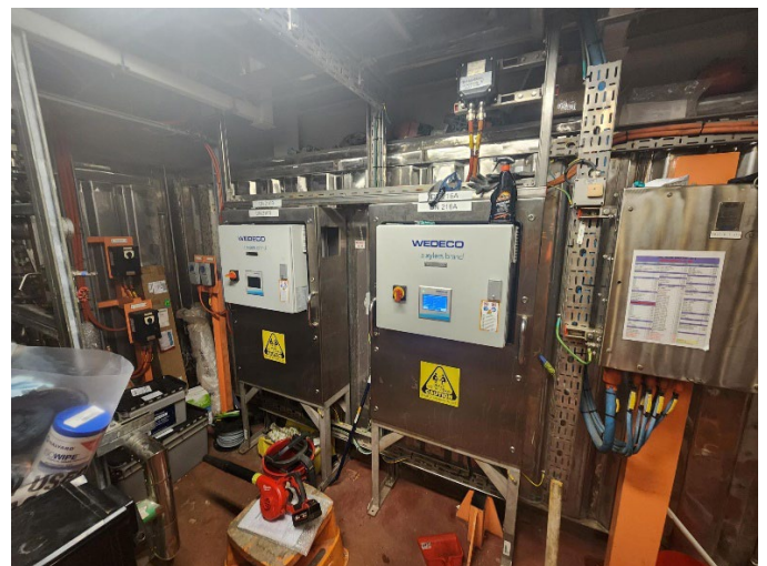
Retrofit control panels in existing cabinets
