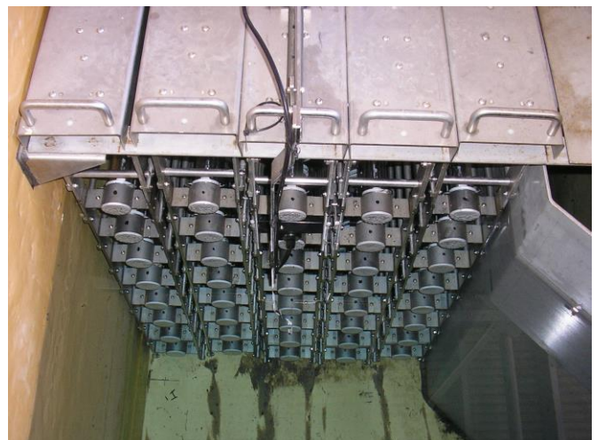
Each bank has 40 lamps, expandable to 56 lamps in future
