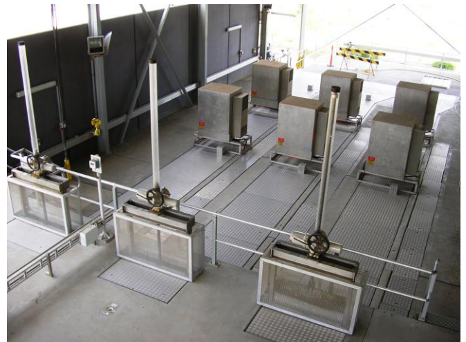
Calgon Carbon UV Technologies C 3 500™D UV system installed at Christies Beach WWTP
