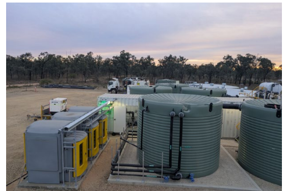
Membrane Bio Reactor (MBR) plant on site
